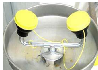
Figure 3. Emergency Eyewash Unit
